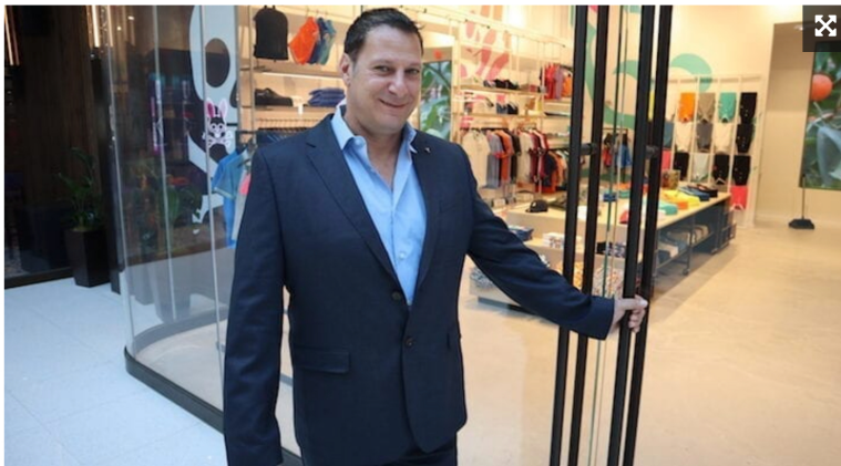
David Vigilante's company, Vigilante Associates, installed 16-foot-by-6-foot glass panels and radius glass panels in the retail area of the Seminole Hard Rock Hotel & Casino in Hollywood, Fla.
